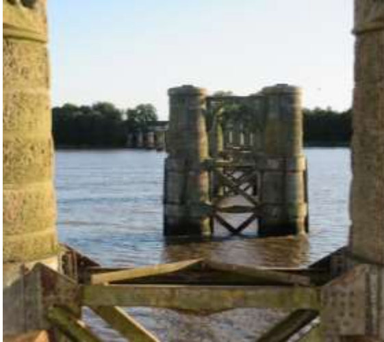
Piers of the bridge. Photo: Nicholas Reid
